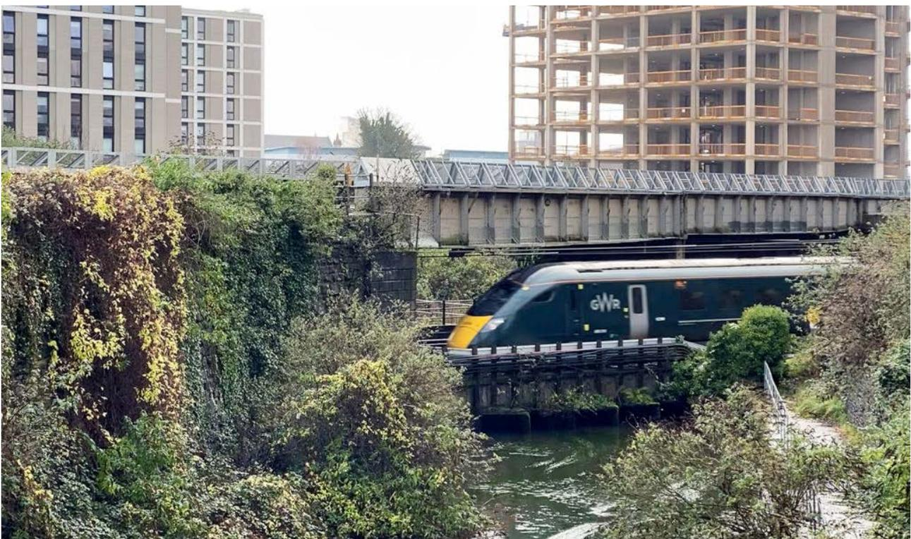
The Intersector Bridge in Cardiff, where new techniques were pioneered to reduce OLE clearances and therefore avoid a very expensive bridge replacement (photograph: © Network Rail)
