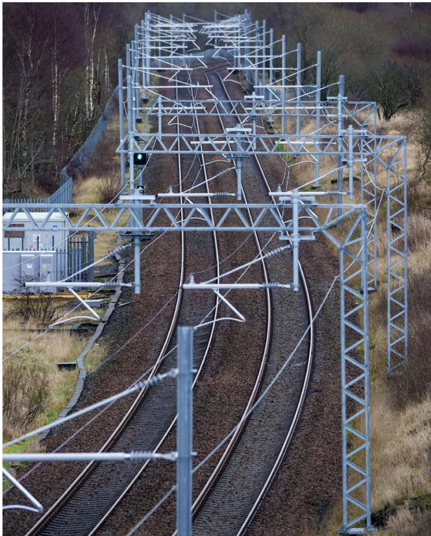
Twin track cantilevers (foreground) and single track cantilevers (background) installed for EGIP (photograph c Network Rail)
