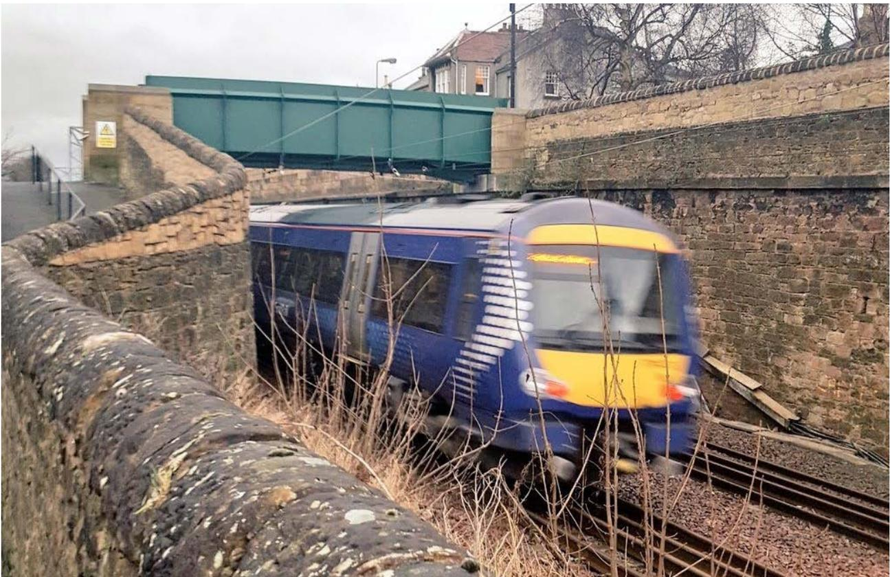
At Linlithgow, boundary walls were sympathetically raised to protect the public from the OLE installed as part of the Edinburgh Glasgow Improvement Programme (EGIP) (photograph: © Network Rail)
