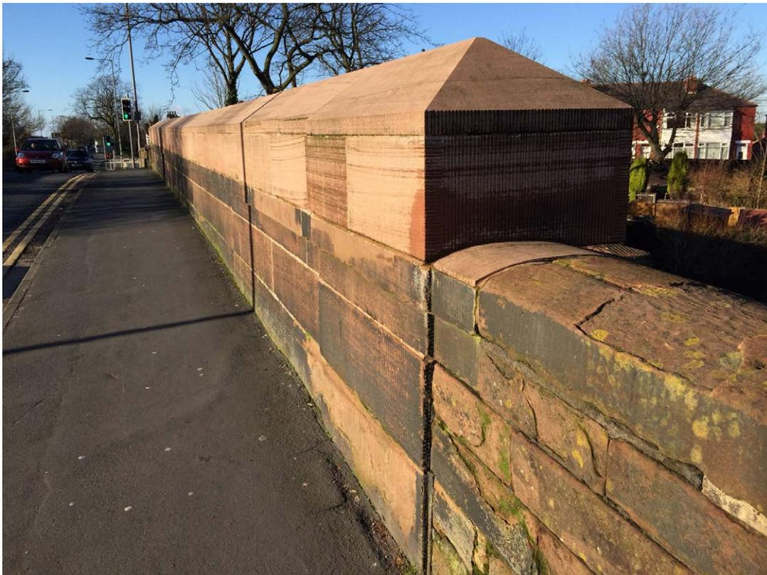
The Rainhill Skew Bridge near Liverpool was designed by George Stephenson as part of the pioneering Liverpool and Manchester Railway in 1830. Recently, the line was electrified and the bridge parapets sympathetically raised. In time, the stone will weather to the same colour (photograph: © Network Rail)
