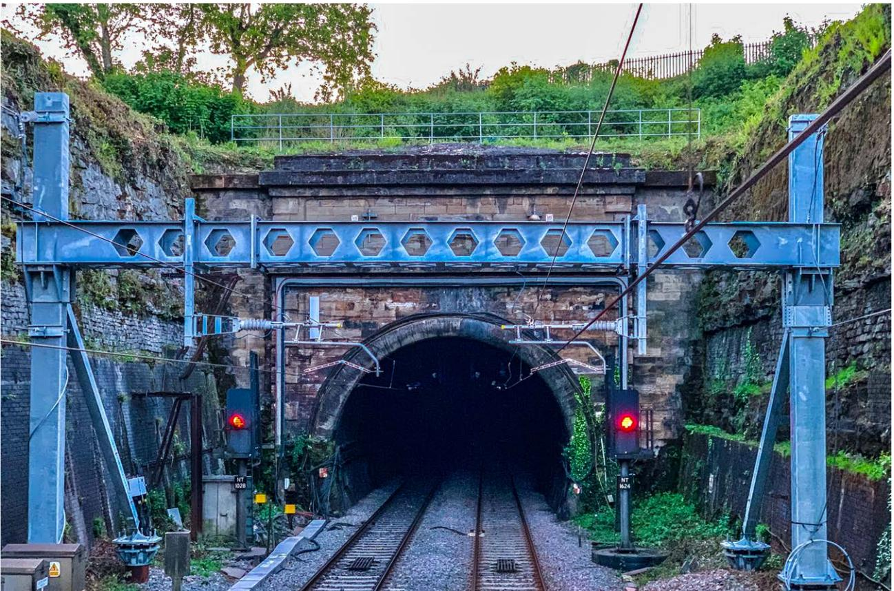
The English portal of the Severn Tunnel (Grade II\*), with OLE installed as part of the Great Western Electrification Programme. The OLE support in the foreground was necessary to avoid attaching the OLE to the stonework of the historic portal (photograph: © Furrer+Freyer)
