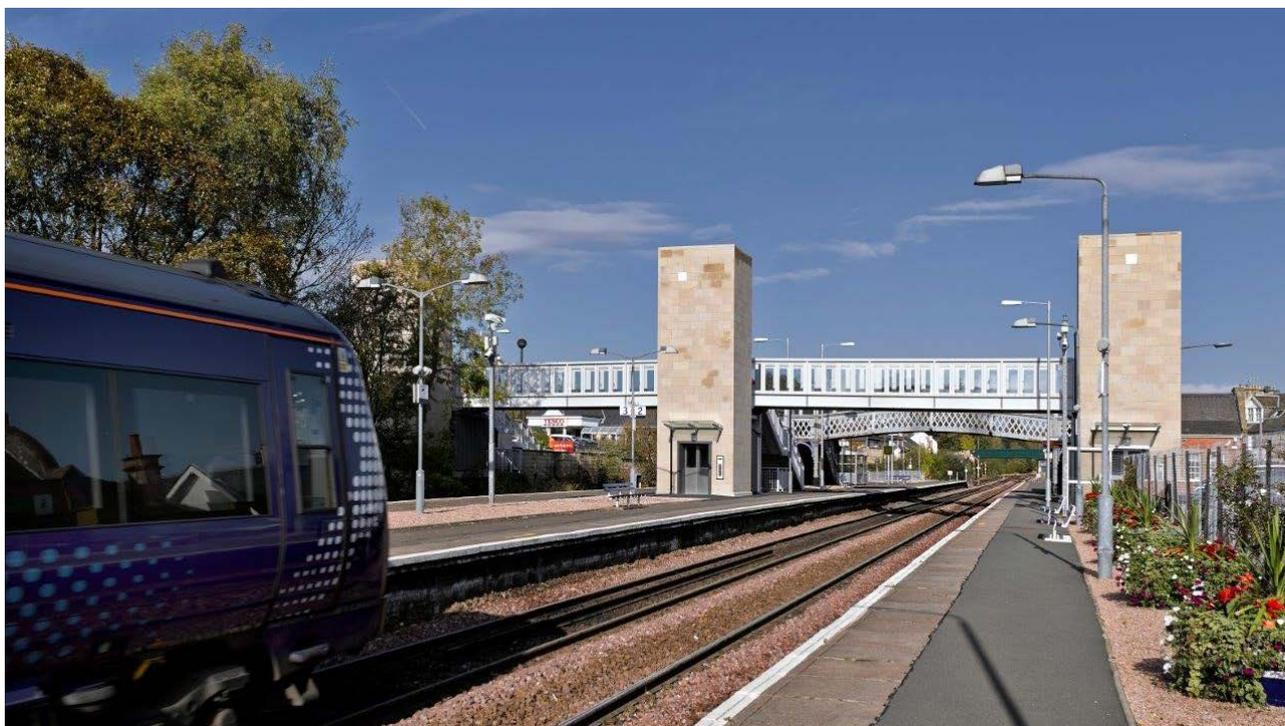
**New level access footbridge at Dunblane Station (Cat B) in place prior to the installation of OLE. The redundant listed historic footbridge in the background has since been dismantled and re-erected for reuse at Bridge of Dun Station on the Caledonian Heritage Railway (photograph: © Network Rail)**
