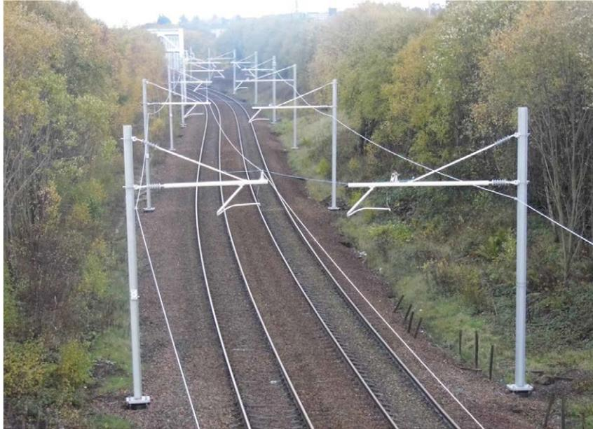
Newly installed UKMS 'single track cantilever' (STC) masts on the Edinburgh Glasgow Improvement Programme (EGIP) (photograph: ©Network Rail)
