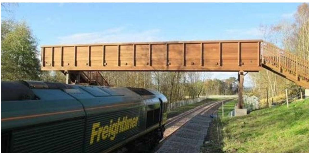
**Timber footbridge installed on the Borders Railway near Gorebridge, where the use of timber helps to blend the bridge with its setting. A similar style bridge has also been used in Princes Street Gardens near Edinburgh Waverley station (photograph: © Network Rail)**
